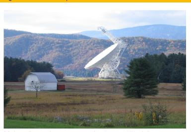
Main reflector is 100x110 m in size, total height 160 m. Entire structure is accurate to 0.25 mm.
