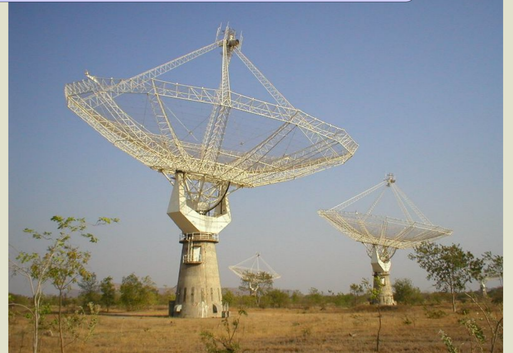
Figure 1: Three of the antennas in the inner square kilometre of the Giant Metrewave Radio Telescope (GMRT). The GMRT consists of 30 antennas in total, each with a diameter of 45 m. Twelve of these are in the inner square kilometre with the remainder distributed in three approximately radial arms extending in NE, NW and S directions. The maximum baseline is approximately 25 km allowing a resolution of 5 arcseconds at 610 MHz.
